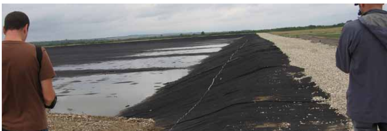
Integrated waste management, Timis (Romania)
