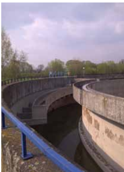
Czechowice - Diecizce wastewater treatment plant (Poland)
