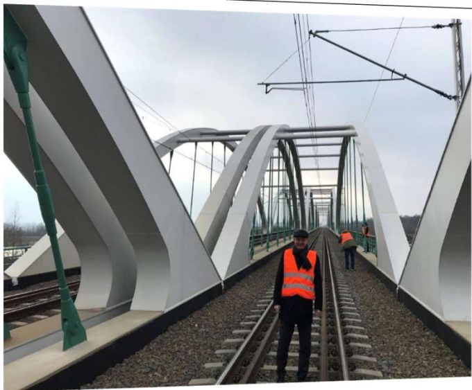
Bridge over Bug river
