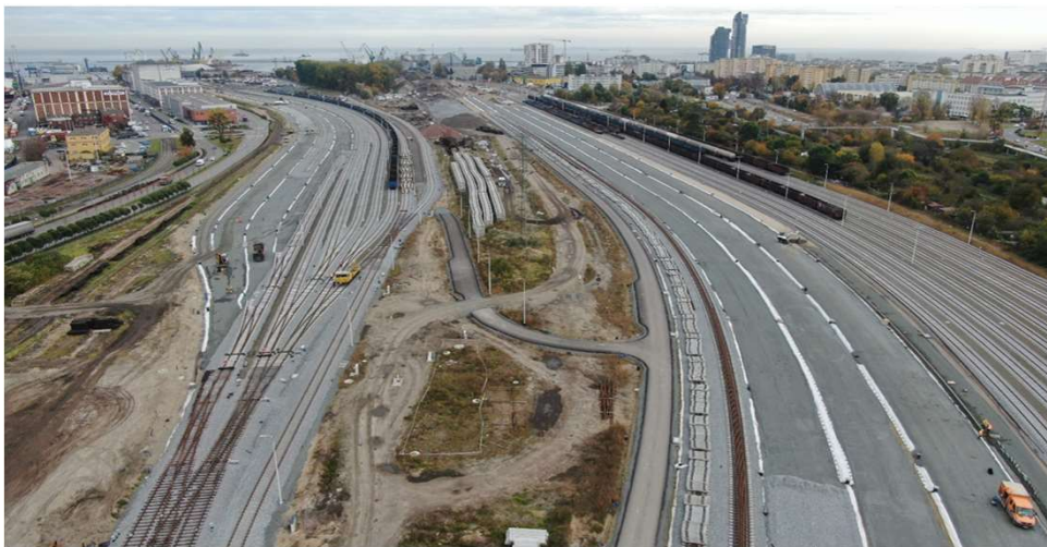
Tracks put into operation in Gdynia
